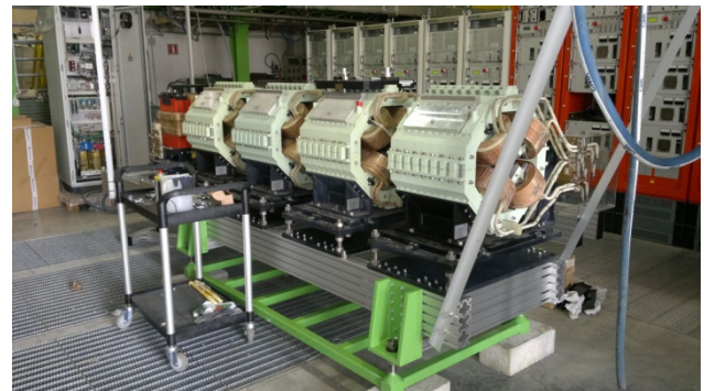
Figure 6: First XPR girder being equipped.
