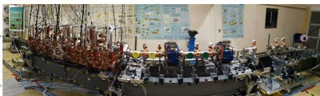
Figure 5: Current status of the installation.
