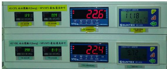
Figure 7: Water pressure/quality/level display module.
