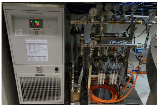
Figure 3: Cooler and water manifold of the HOM water-cooling system.
