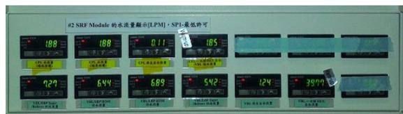
Figure 5: Water flow-meter module.
