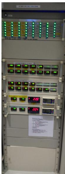
Figure 2: Electronic rack of the TPS superconducting cavity CPL/HOM water-quality and cooling system.
