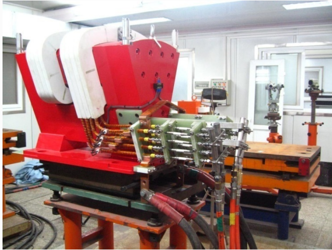
Transport line dipole
