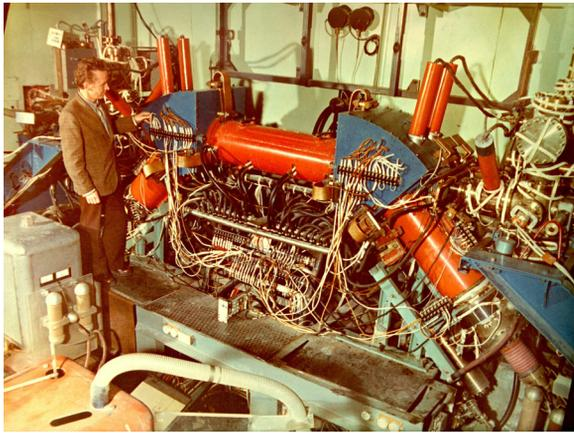
Figure 1: The first electron cooling installation in the NAP-M storage ring.
