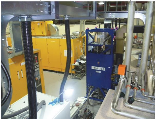
Figure 2: 300kW klystron and KSU of RF system.
