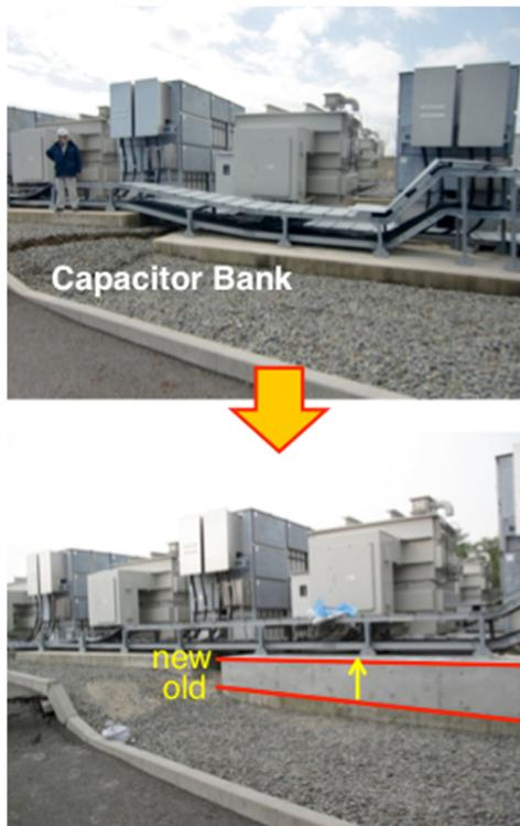
Figure 6: Around 3 GeV a significant amount of concrete shield had to be added to bring it to the normal level.
