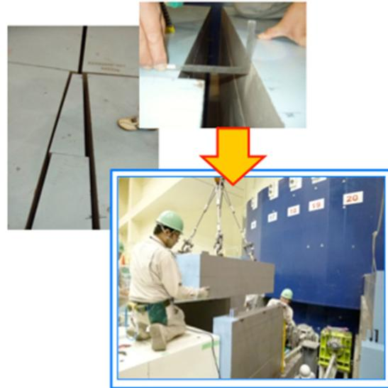
Figure 7: Movement of ion shield. 2,800 tons of irons have to be removed and restacked.
