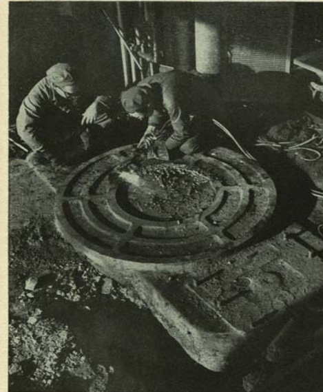
BASE OF CYCLOTRON, which was imbedded in concrete, is defaced by acetylene torch so it cannot be used again. Magnet's huge copper coils were lifted out by cranes.
