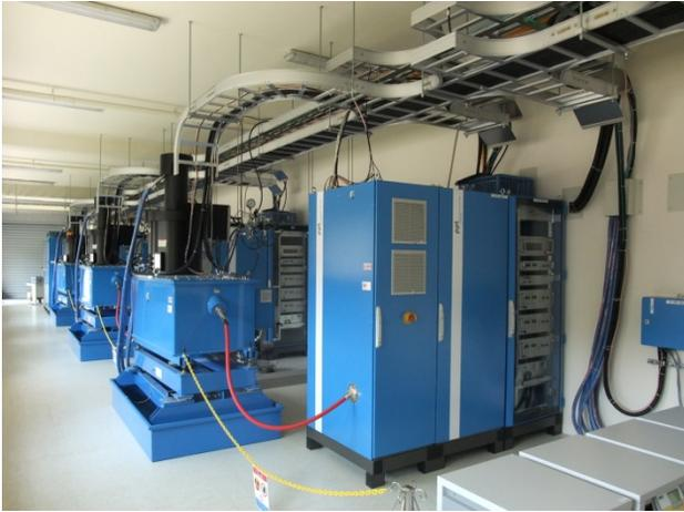
Figure 2: The linac rf stations.
