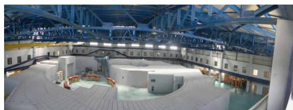
Figure1: SESAME Radiation shielding wall.
