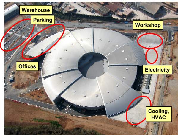
Figure 1: A picture of the ALBA-Building
