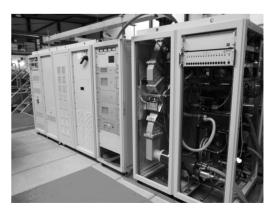
Figure 3: 30 kW IOT based transmitter
