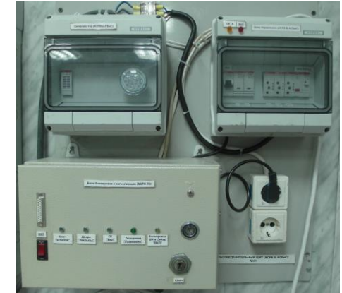
Interlocking and alarm system switchboard
