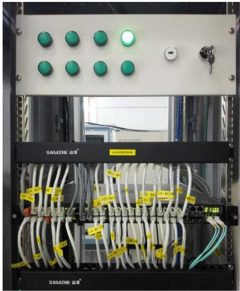
Figure 3: The design of control panel for mode selection.
