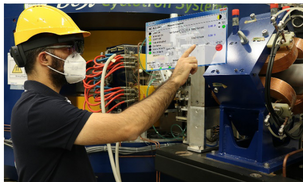
Figure 3: Preliminary tests with AR technology for maintenance operations.
