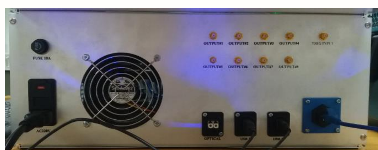
Figure 3: Installation of the hardware.
