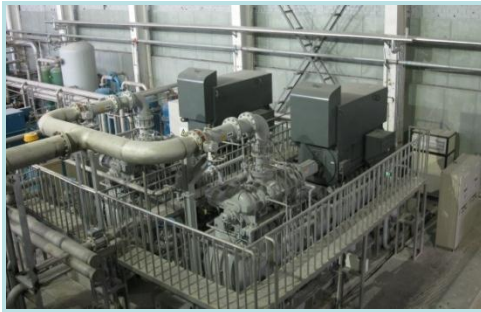
Warm Compressor Station & 10000 Nm 3 helium gas tanks
