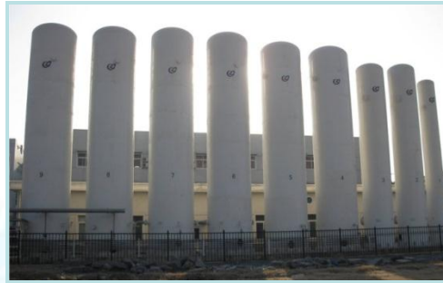
Warm Compressor Station & 10000 Nm 3 helium gas tanks
