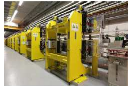
> FLASH2 variable gap undulators
