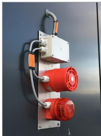
Figure 7: Alarm plate installed in the facade of the HCB.
