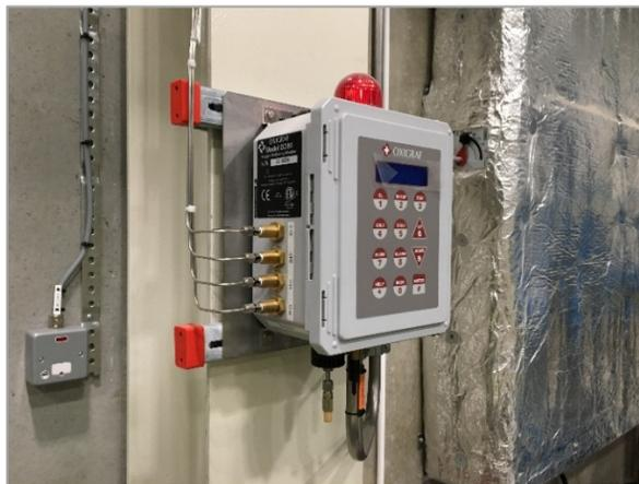
Figure 4: O2iM 4-port mounted in a pillar at the HCB.
