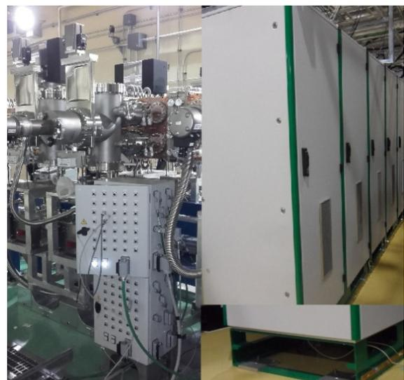
Figure 4: RFQ LCS junction boxes (on the left) and cubicles (on the right).
