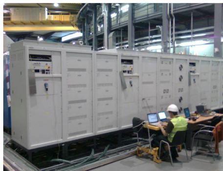
Figure 1: Main Booster Power Supplies during commissioning
