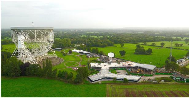
Figure 1: Aerial view of the current status of the SKAO HQ2 building, after the steel structure has been erected, and concrete slabs installed. The current SKAO HQ is in the foreground, Council chamber can be seen raising to the right.
