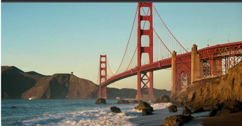
Golden Gate Bridge
