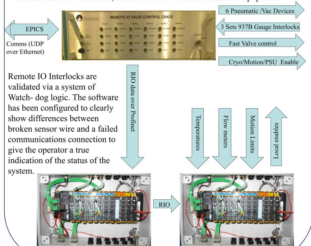
Remote IO Interlocks are validated via a system of Watch-dog logic. The software has been configured to clearly show differences between broken sensor wire and a failed communications connection to give the operator a true indication of the status of the system.
