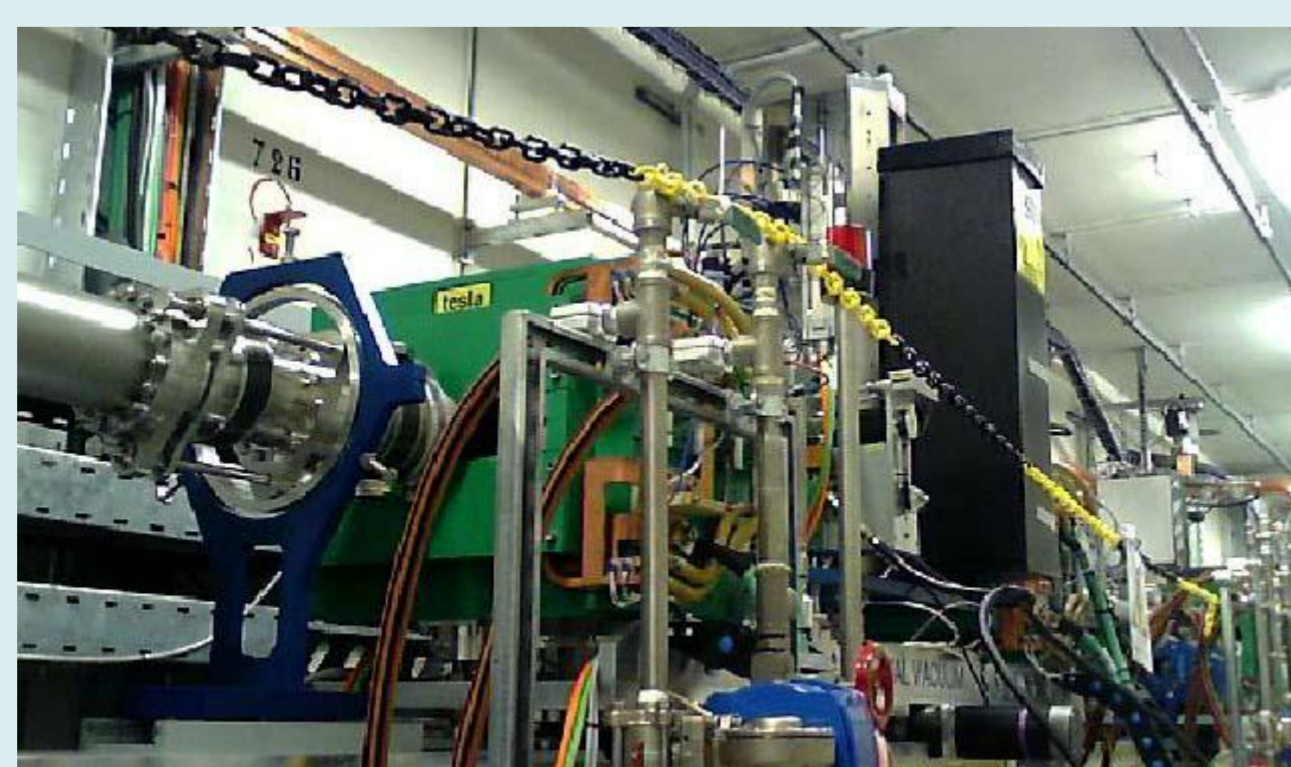
Bunch Compressor, an heavy duty installation.
