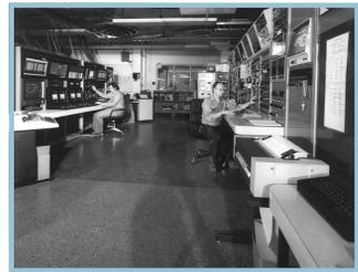
The right side of the room is the original (not computer controlled) control of the accelerator.
