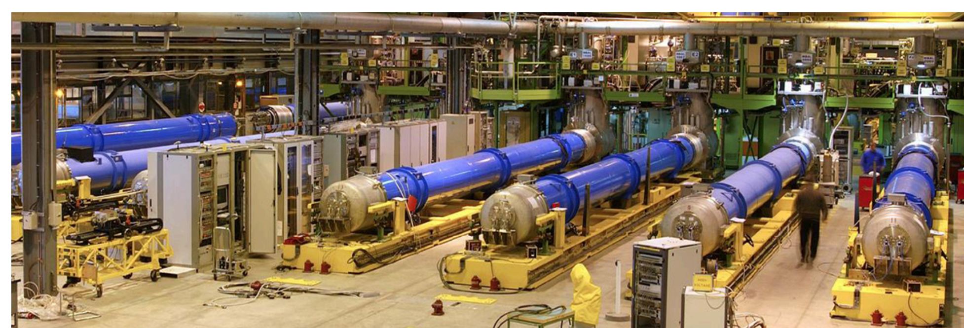
View of half of the SM18 test benches facility.
