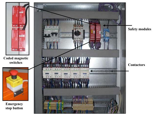
Figure 3: The LASER safety control system.
