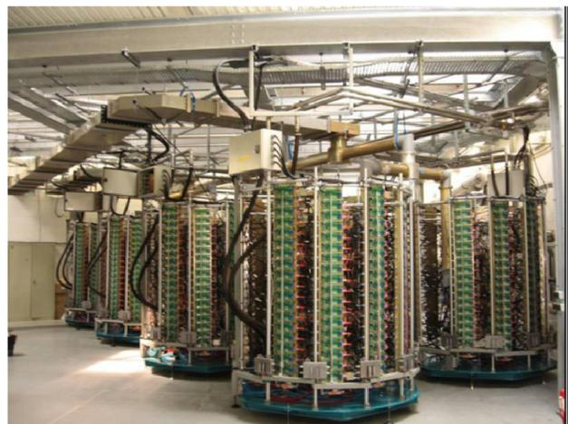
Figure 7: Solid state RF amplifier at Soleil.
