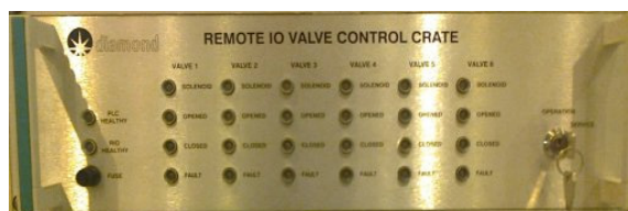
Figure 2: PLC sub system for control vacuum valves.
