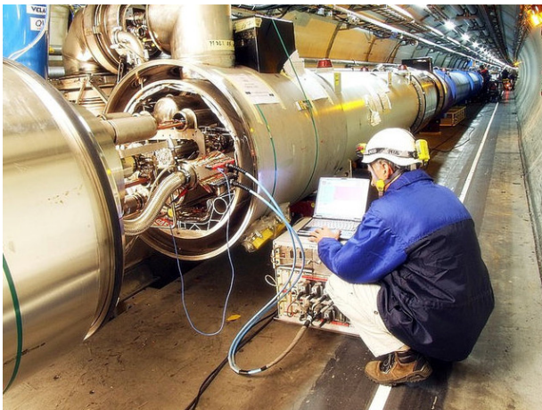
Figure 2: High Voltage qualification in the LHC tunnel.
