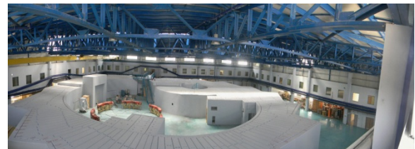
Figure 1: SESAME radiation shielding wall.
