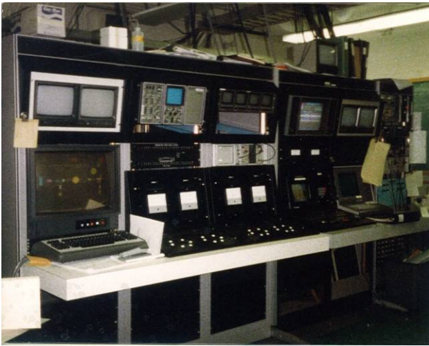
Figure 3: Control Room circa 1985. The right (grey counter) is the accelerator control system including the original Booster and added ATLAS sections. The left (white counter) is the added beamline control system.
