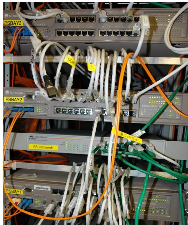
Figure 2: Different flavour of network switches running in HIPA Controls network until the end of 2010.
