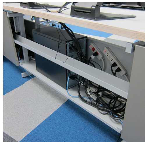
Figure 3: Back view of the control desk. A workstation is built in. Two lines of AC power are supplied. One is stabilized by UPS for the workstation and the other is not stabilized.
