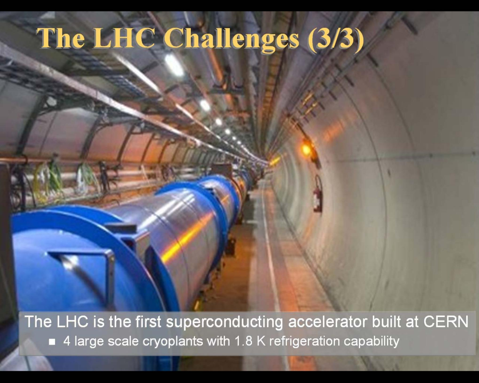
The LHC is the first superconducting accelerator built at CERN
