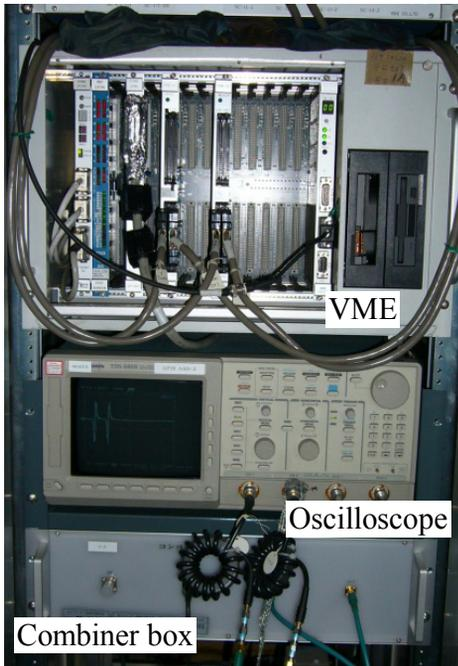
Figure 2: Photograph of previous BPM DAQ system.
