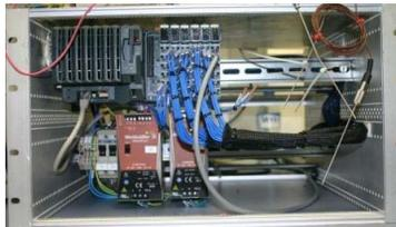
**Figure 4: B&R PLC for vacuum interlocks installed in a rack in the Service Area.**
