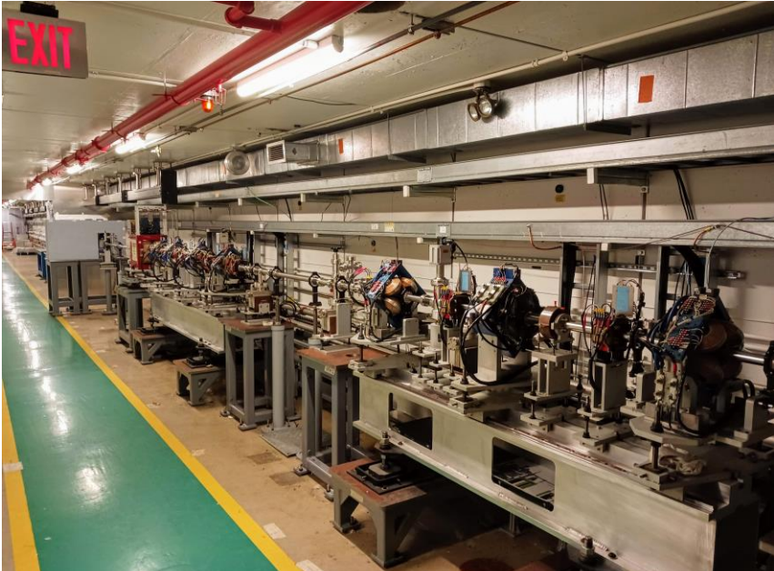
Fig. 3: Photograph of the LEA beamline within the LEA enclosure. In this figure the beam direction is from right to left.
