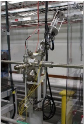
Profile monitor in Linac Segment (LS3)
