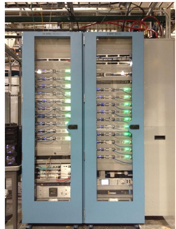
Storage Ring Thermal Racks Regulated to \pm 0.1^\circ\text{C}
