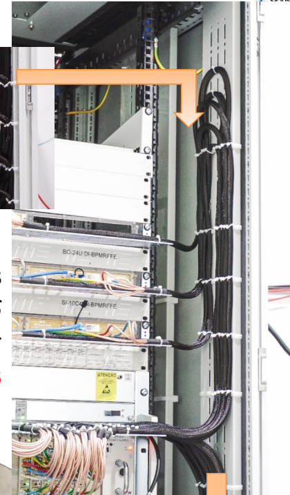
Intra Rack Cables Double shielded RG316 RFFE output → Digitizer 2 meters
