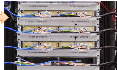
Intra Rack Cables Double shielded RG316 RFFE output → Digitizer 2 meters
