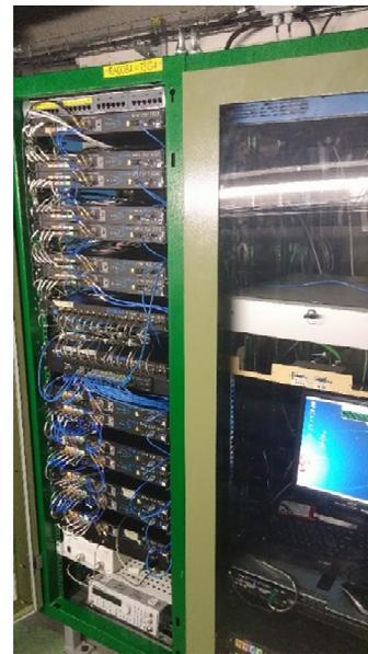
Figure 4: BPM DSP rack and TRIUMF Linux PC.
