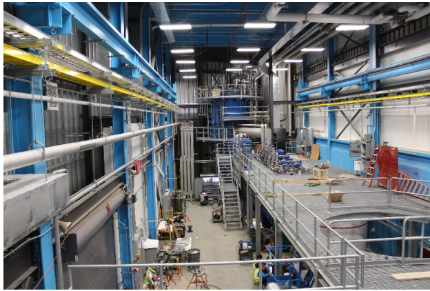
Figure 6: 4.5 K coldbox installed in the FRIB cryogenics building [9]. The Floating Pressure Process – Ganni Cycle [10] is implemented to provide efficient adaptation to the actual loads.
