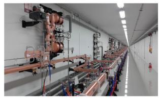
Figure 2: Accelerating structures inside the PAL-XFEL linac tunnel.
