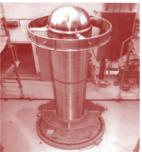
Figure 4: CN Van de Graaff accelerator operated at 5.5 MeV at IRN in 1959. Coaxial ring electrodes installed along acceleration column with terminal at the top.
