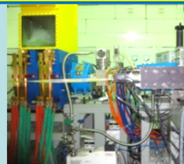
EV cooling LECR4 2010-2014
