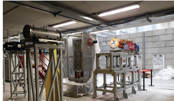
Figure 4: Charge Breeder installation.
