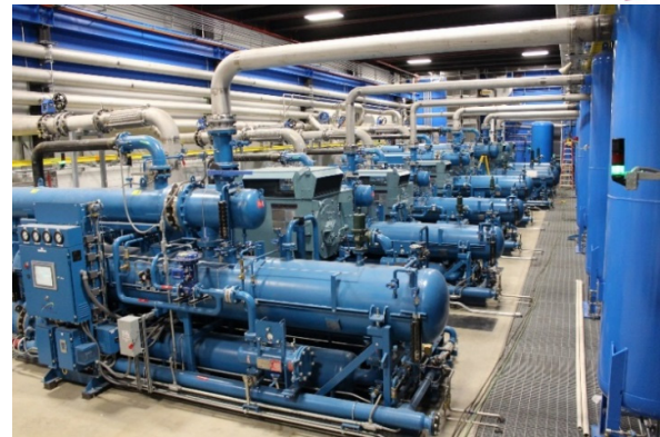
Figure 10: Cryoplant compressors located in the FRIB building (bottom) and the measured tunnel vibration (top).
