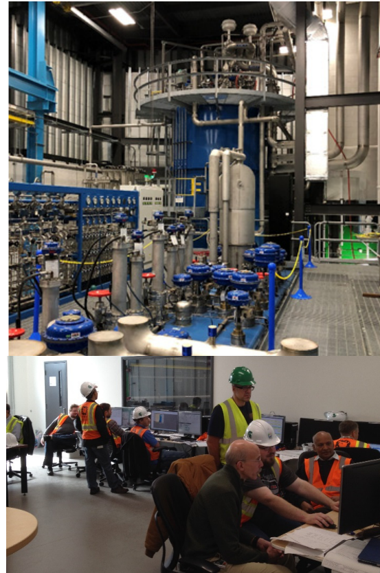
Figure 4: Commissioning of the FRIB cryoplant at 4 K.
