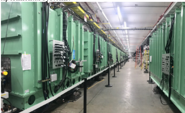
Figure 6: Cryomodules installed for ARR3 commissioning.
