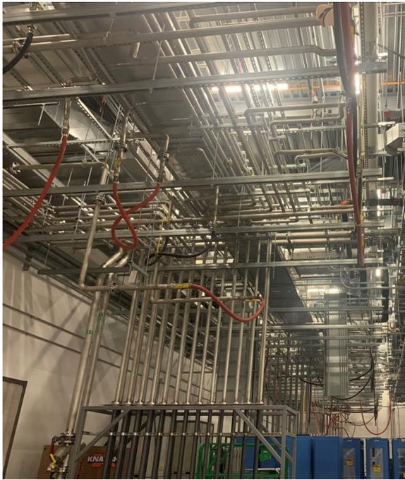
Figure 6: Klystron gallery installed cooling systems.
