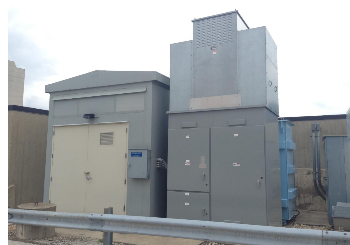
SS Driver - Modulator - Bias supply
