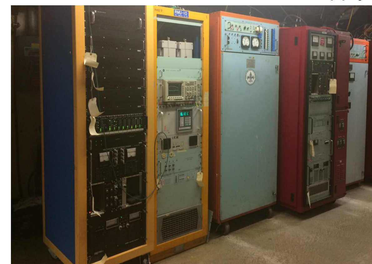
SS Driver - Modulator - Bias supply
