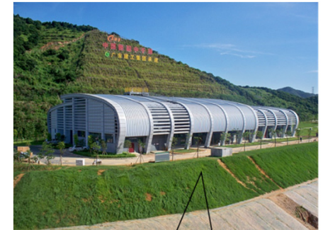
The Linac RF power sources hall
